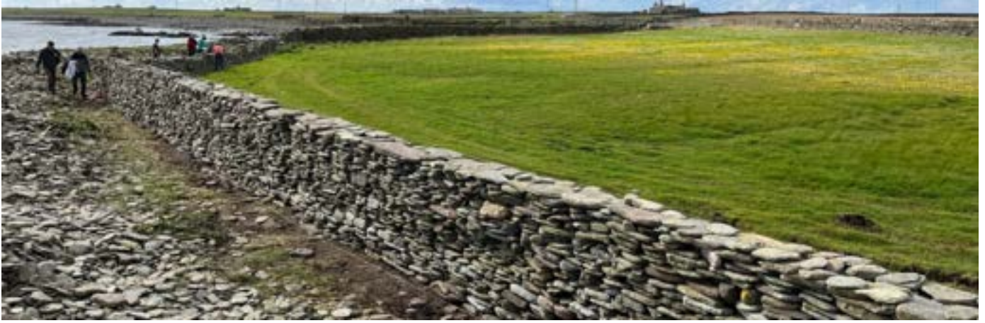
Completed Sheepdyke at Bewan
