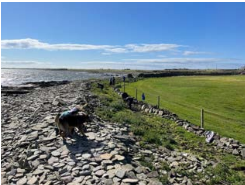
The dyke at Bewan before work began
